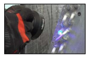
**NOTE:** Do not bend, cut or deform EasyDye tube. Be careful not to allow refrigerant to spray on bare skin, as it could cause frostbite.
